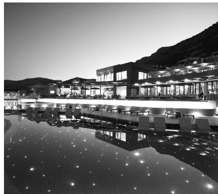
DELTA ELECTRICAL DERMITZAKIS Cayo Resort and Spa
