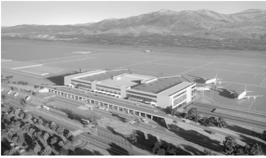
DELTA DUCT DERMITZAKIS New Airport of Crete
