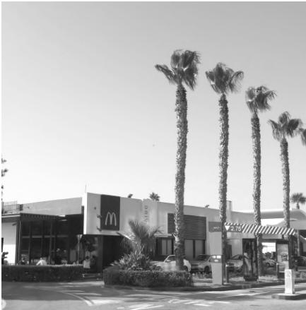
DELTA DUCT DERMITZAKIS Mc Donald's Malta & Romania
