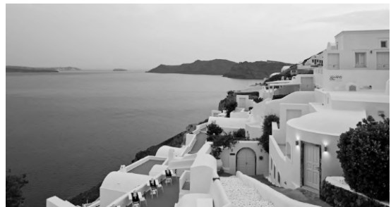
DELTA DUCT DERMITZAKIS Canaves Oia Santorini
