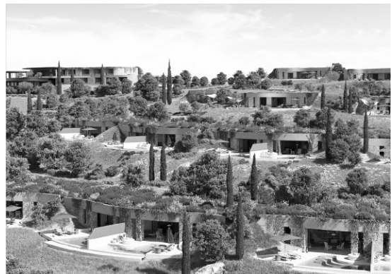
DELTA DUCT DERMITZAKIS Costa Navarino
