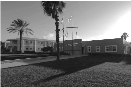
DELTA DERMITZAKIS Communication Station, NSA Souda
