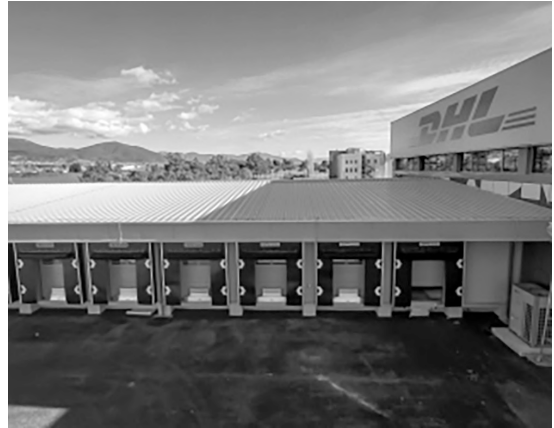
DELTA DUCT DERMITZAKIS Projects Redex AE
