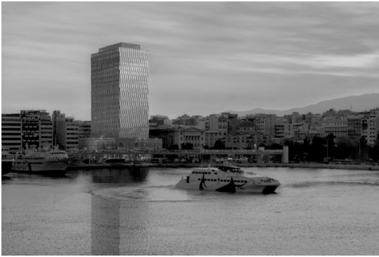
DELTA DUCT DERMITZAKIS Zara Store, Piraeus Tower
